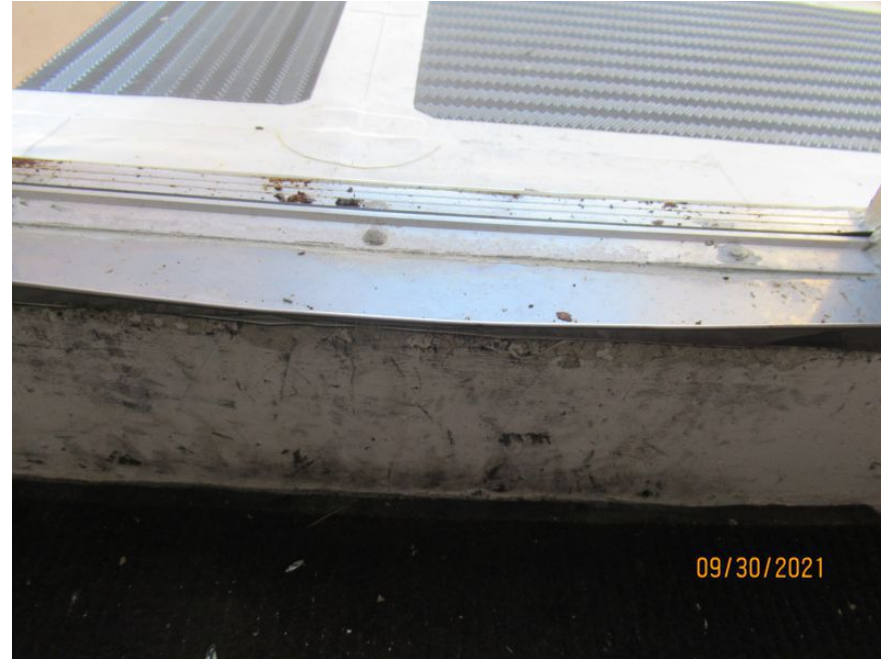
Reinforced Concrete Roof Deck
